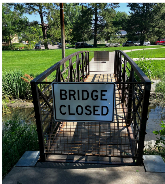
Existing pedestrian bridge.
